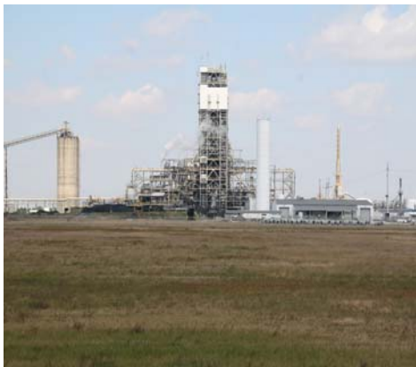
Single tower gasification plant located in Florida. Lake Charles Cogeneration proposed plant at the Port of Lake Charles calls for a five (5) tower gasification plant.
